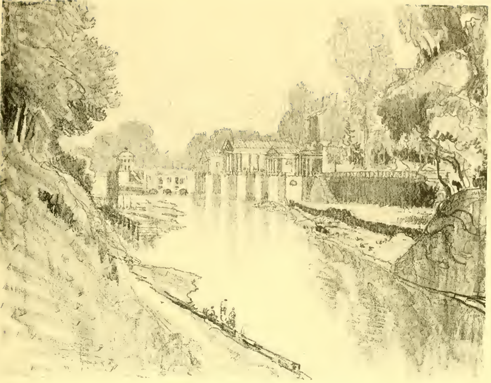
THE BASIN, OLD WATER-WORKS
